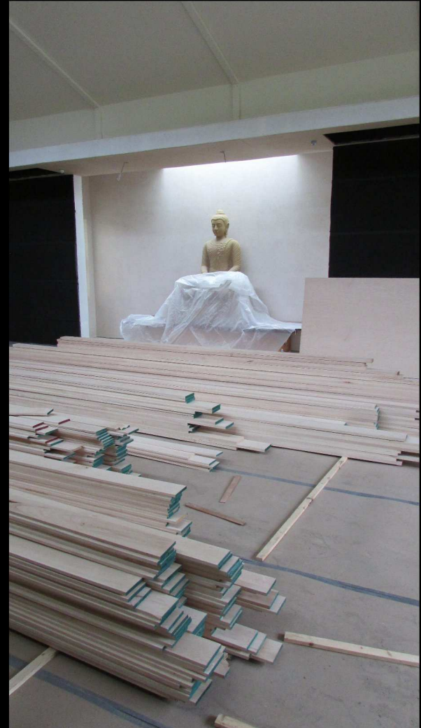
Reception hall is still a construction site
