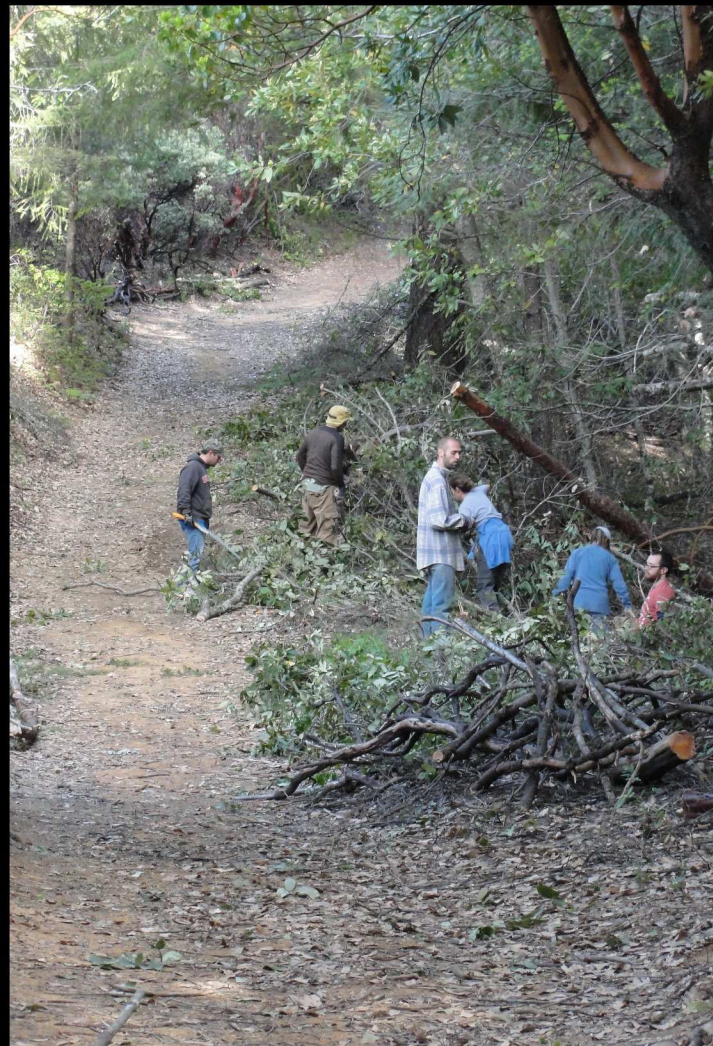
Widening our road
