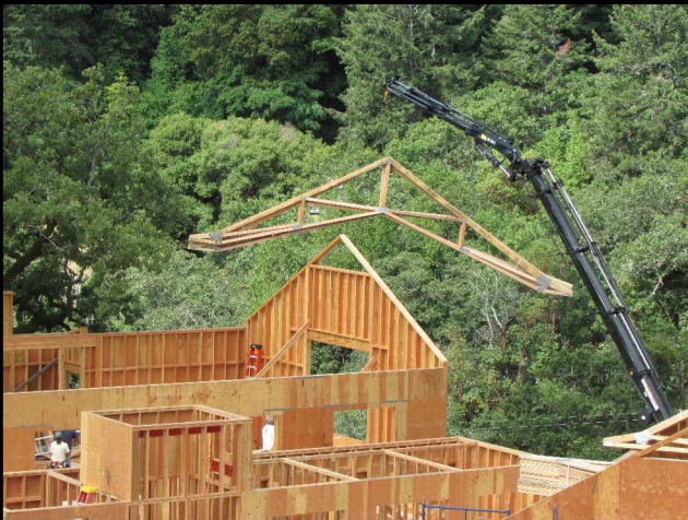
Roof trusses going on meditation hall.
