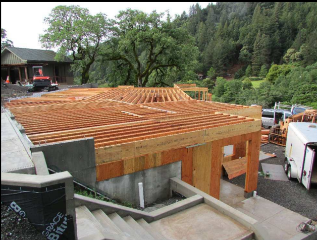
2nd story floor framing complete.
