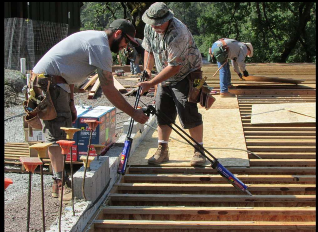
Glue bonding floor boards on.
